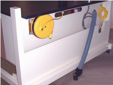
Rear chase area showing service and equipment 'quick' connections
