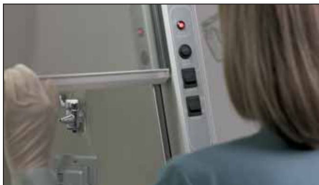
Controls are mounted in the user's field of vision to limit neck movement and meet ADA requirements.
